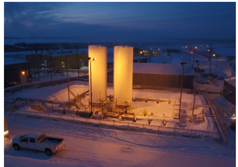
Figure 23 NTPC's Inuvik LNG Storage Facility
